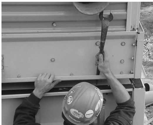
Figure 4. Drift Pin Alignment
