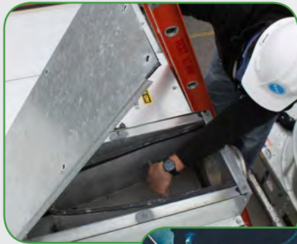
Inlet strainer inspection for Series 1500
