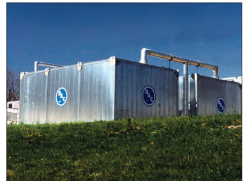
Modular Ice Thermal Storage Unit
