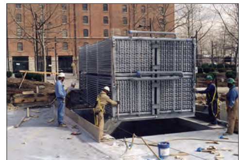
BAC ICE Coil Installation Camden Yards
