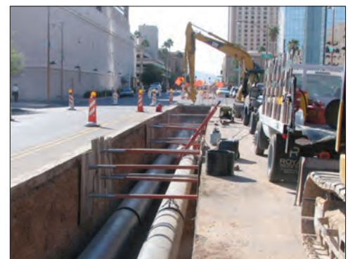
District Cooling Piping Installation
