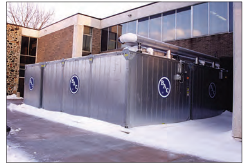
TSUM Installation Catonsville Community College
