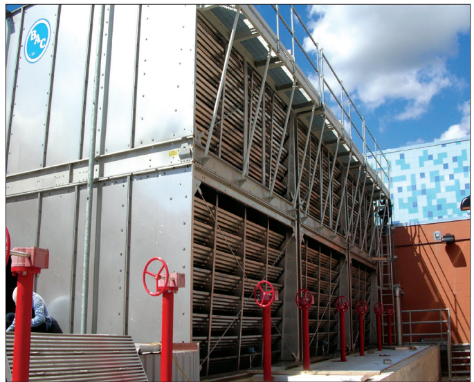
Three Cell Installation on Concrete Basin
