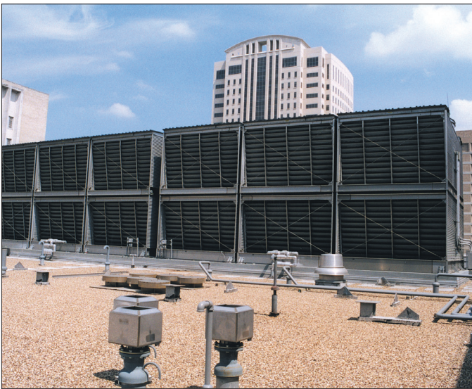
Six Cell Installation on Concrete Basin
