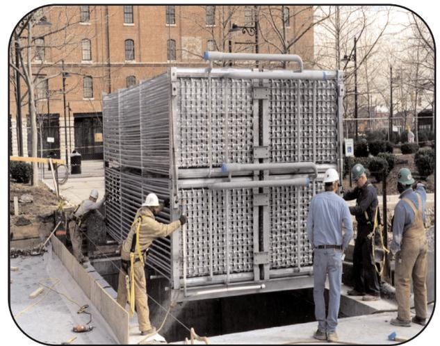
Rigging ice coil into underground vault
