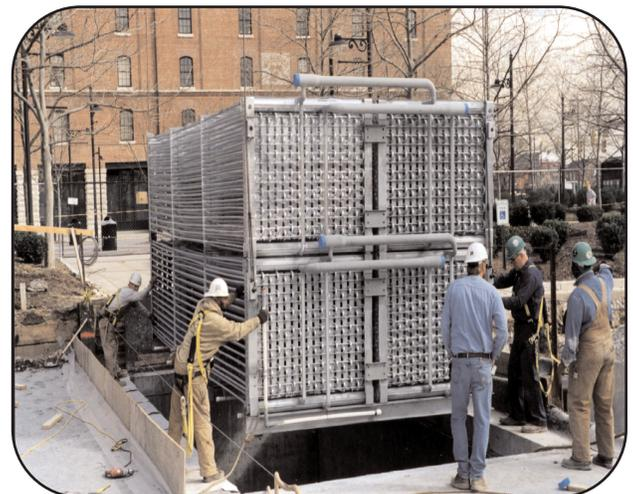
Rigging ice coil into underground vault
