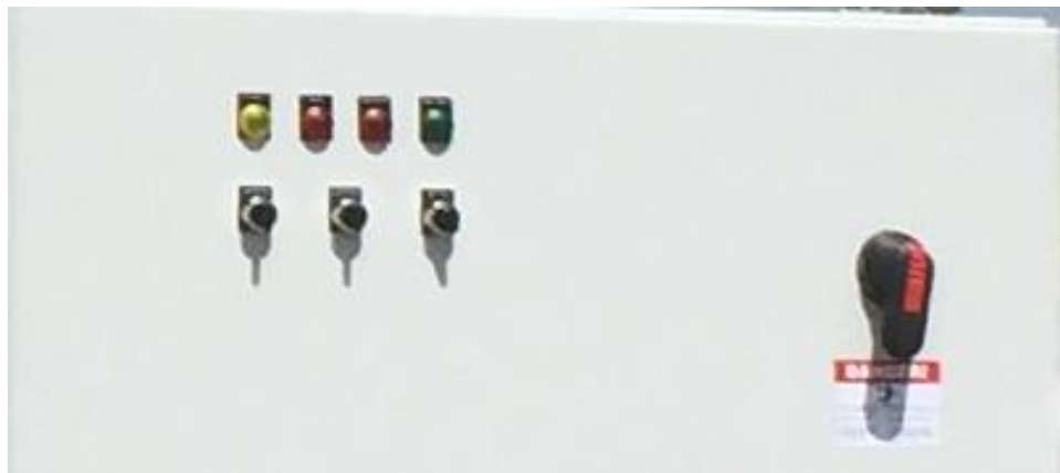
VFD Only Enclosure
