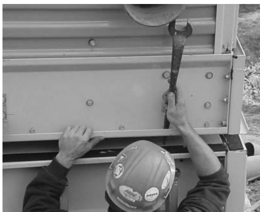
Figure 4. Drift Pin Alignment
