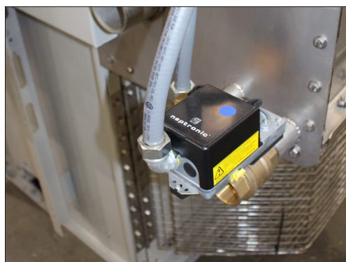
Figure 21. Drain Valve
