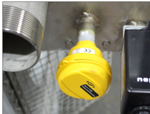
Figure 30. Conductivity Sensor
