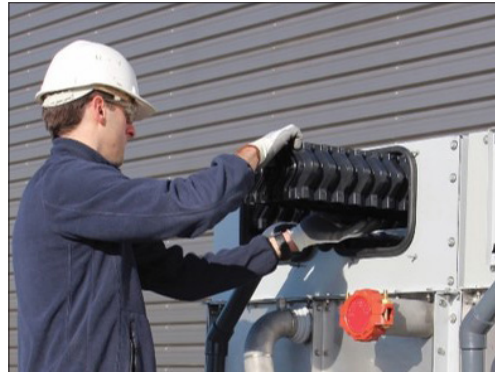
Figure 25. Drift Eliminator Removal
