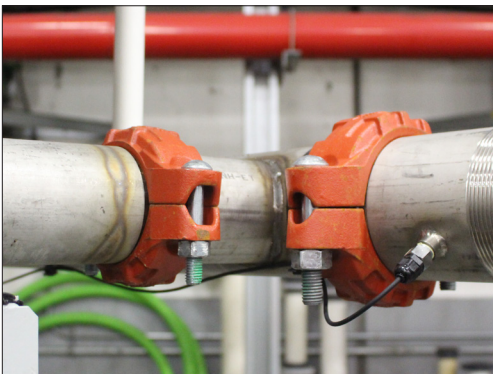
Figure 28. Leaving Process Fluid Temperature Sensor
