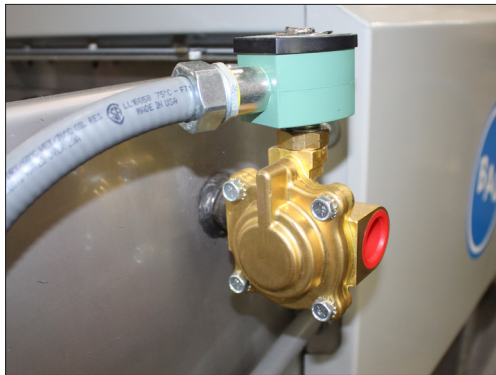
Figure 27. Solenoid Make-up Valve
