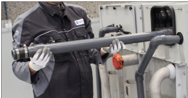
Figure 24. Spray Branch Removal
