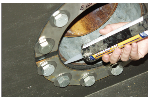
Figure 14. Caulk Exposed Galvanized Steel
