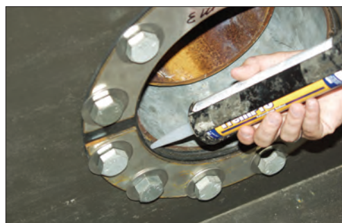
Figure 17. Caulk Exposed Galvanized Steel
