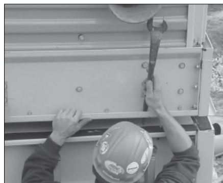
Figure 5. Section Alignment Using Drift Pins
