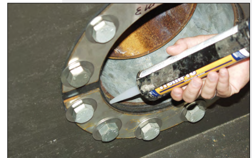
Figure 17. Caulk Exposed Galvanized Steel
