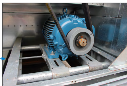
Figure 4. Motor Adjusting Screw
