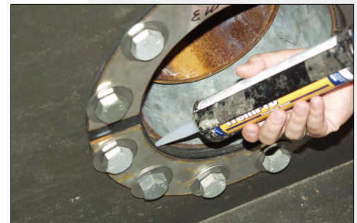
Figure 22. Caulk Exposed Galvanized Steel
