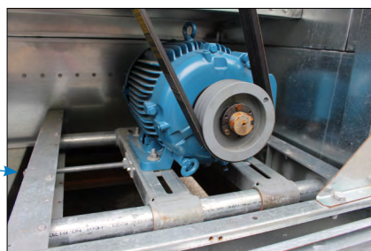
Figure 4. Motor Adjusting Screw
