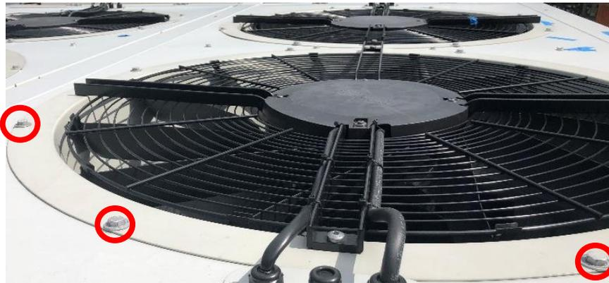
Figure 18. Fan Deck Fasteners
