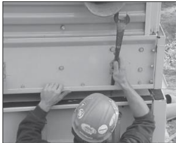
Figure 4. Section Alignment Using Drift Pins
