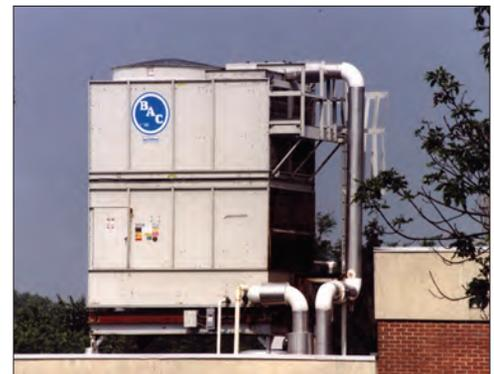
Thermosetting Hybrid Polymer Construction Installation
