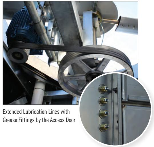
Extended Lubrication Lines with Grease Fittings by the Access Door
