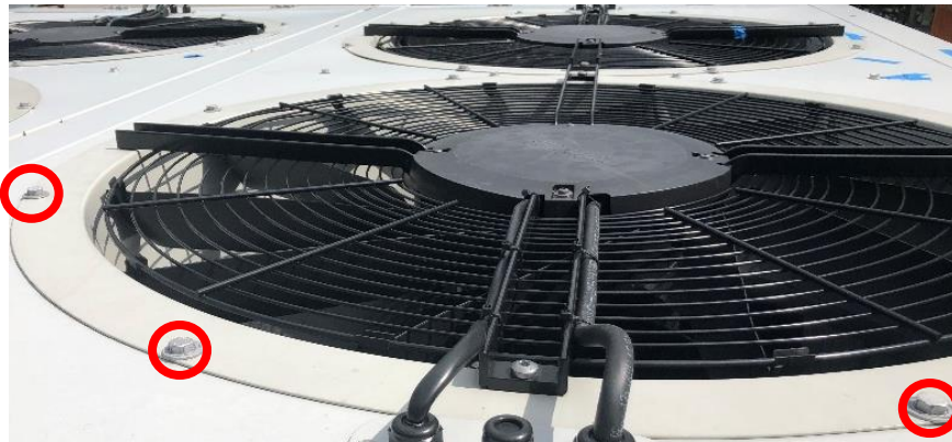
Figure 18. Fan Deck Fasteners
