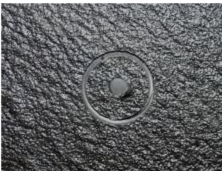
Figure 23. Scored TriArmor® Corrosion Protection System
