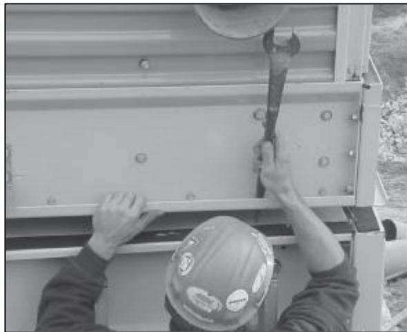
Figure 4. Section Alignment Using Drift Pins
