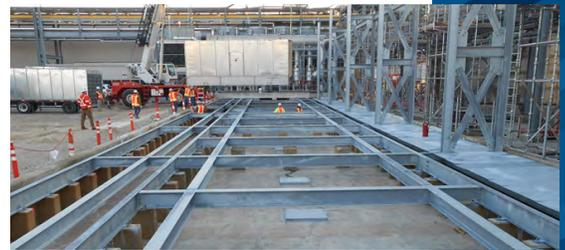
The BAC Series 3000 modules were installed on the existing concrete cold-water basin
