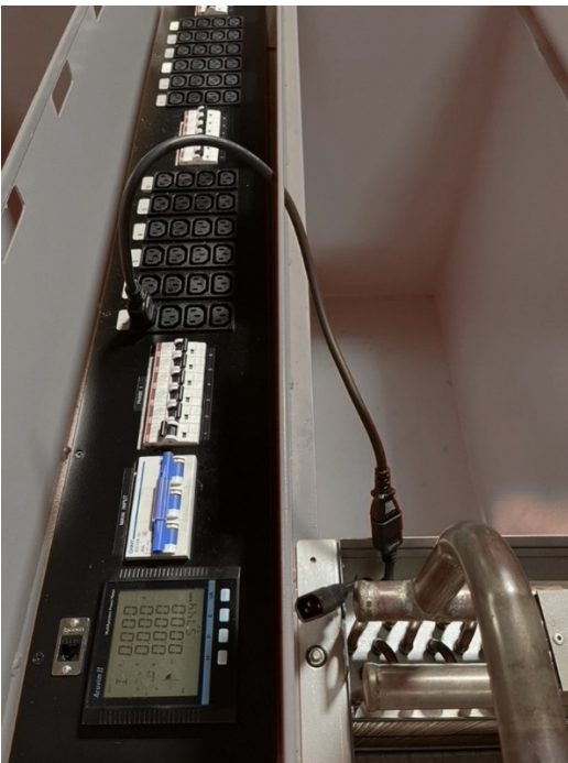
Figure 33: One of two FCM pumps plugged in using extension lead connected to PDU, ready for bump testing
