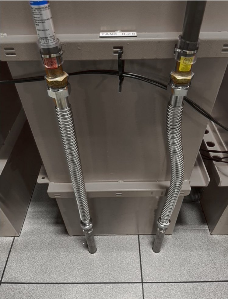
Figure 22: Flexible hoses (not supplied) connecting the FCM's cooling water inlet and outlet to the cooling water loop
