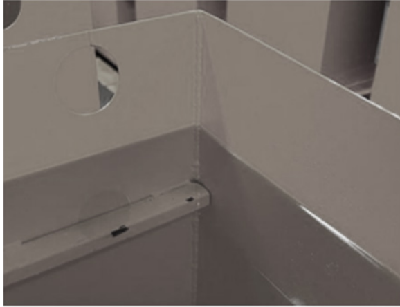
Figure 36: Tank initially filled at a high level for leak testing before level reduction and installation of servers
