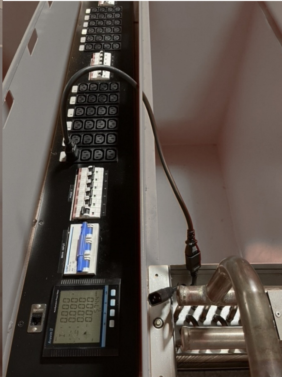
Figure 30: An extension cable running from the PDU to one of the two FCM pump power cables
