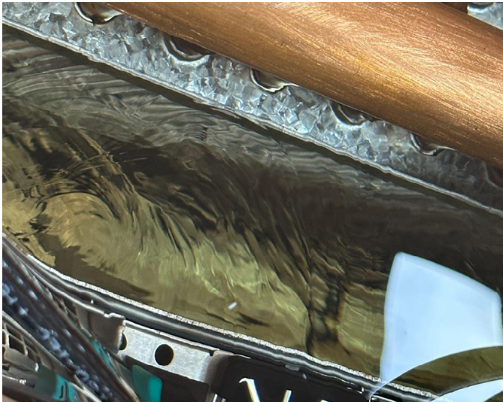
Figure 38: Close up of vortex in immersion cooling fluid indicating that pumps are running.
