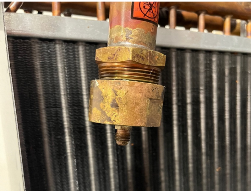
Figure 21: FCM cooling water inlet and outlet fitted with end caps with Schrader valve
