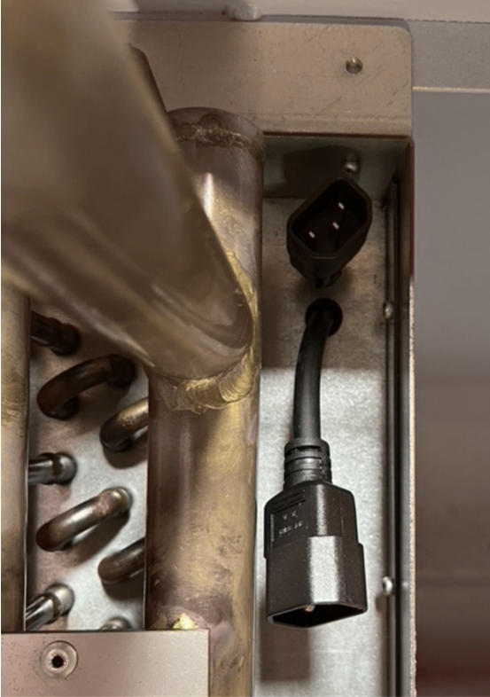
Figure 29: Two FCM pump power cables on top of FCM, before connection of extension cables
