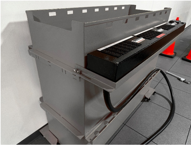
Figure 31: Tank with PDU bracket and PDU installed
