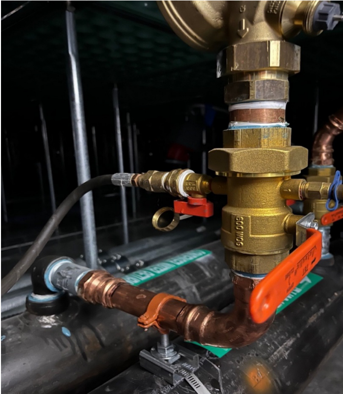
Figure 25: Hydrostatic pressure tester attached to tap in valve to pressurize the FCM circuit. Note the black hose connected.
