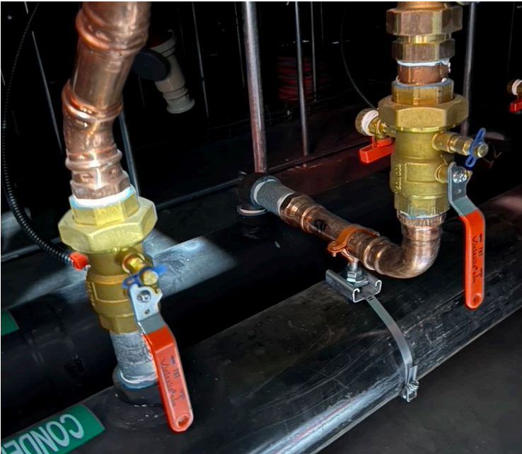
Figure 27: Both inlet and outlet shut off valves are open, with testing equipment removed and caps reinstalled
