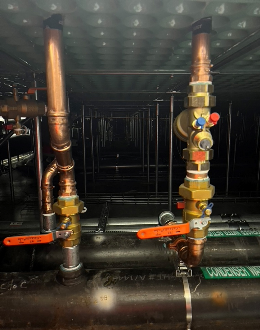
Figure 23: Example of cooling water circuit with both shut off valves visible in closed position
