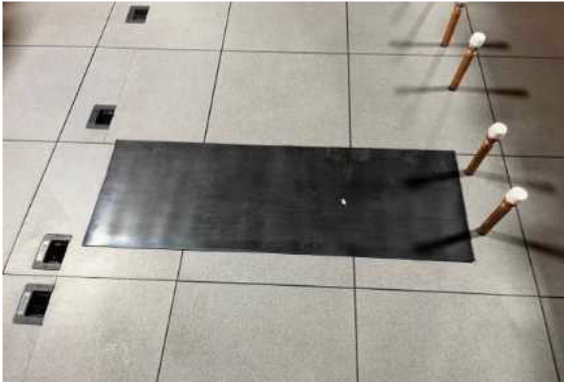
Figure 10: Rubber mat positioned on floor before tank installation
