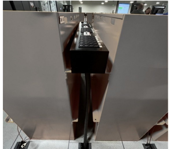
Figure 32: PDU on support ledge between two tanks, not using PDU bracket
