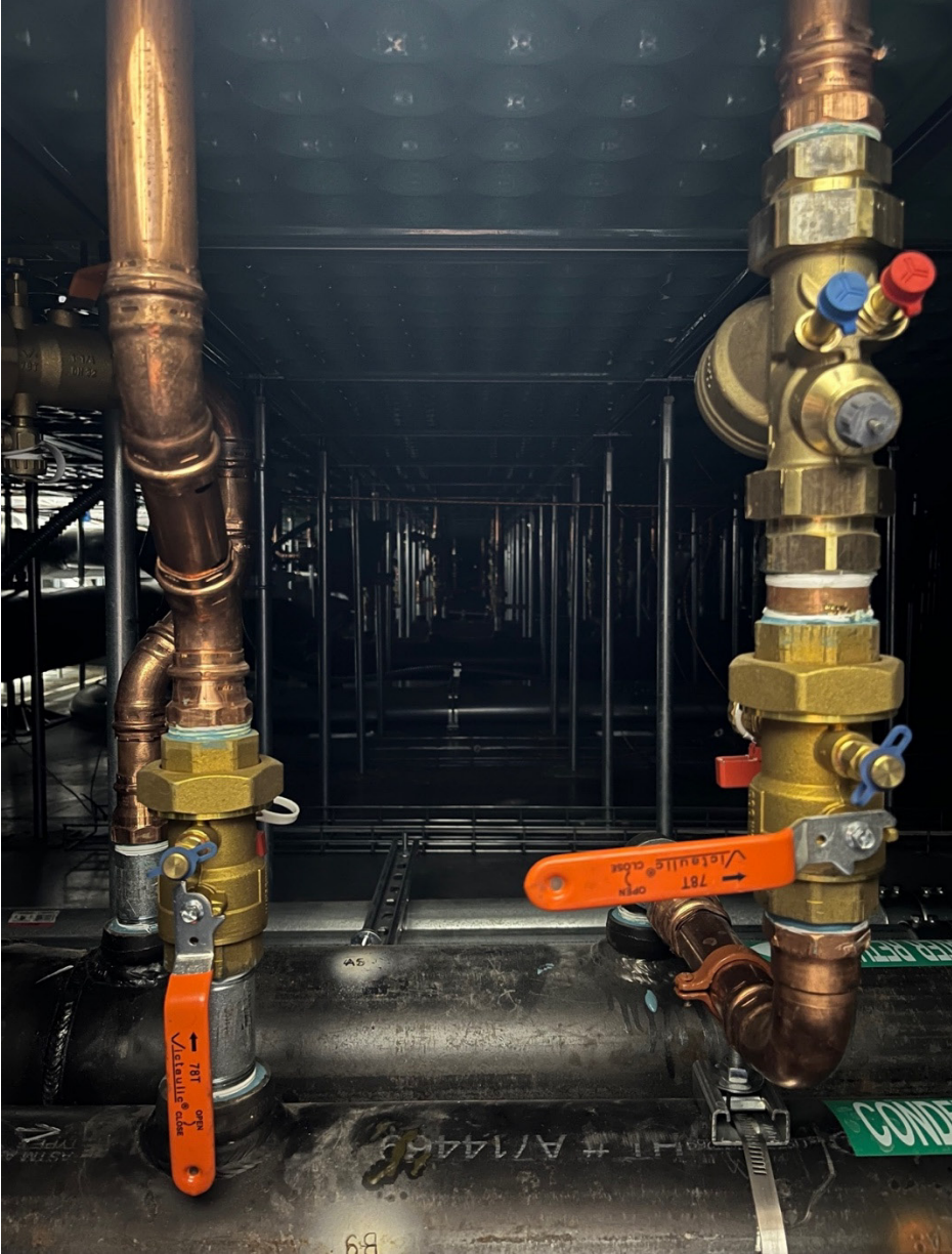
Figure 24: Example of cooling water circuit with inlet shut off valve open (on left), and outlet shut off valve in closed (on right)
