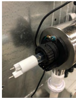
Figure 49. UV Bulb connection
