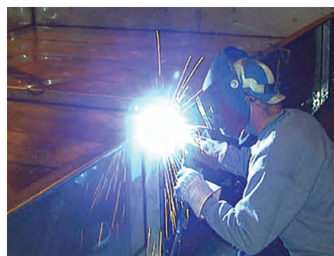
Welded Stainless Steel Cold Water Basin
