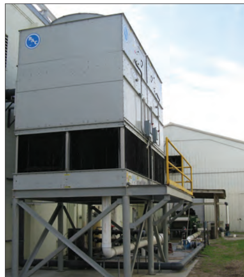
EVERTOUGH™ Construction Installation
