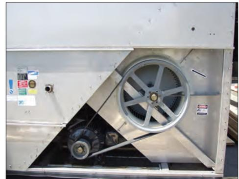
Moving Parts Located Near Base of Unit
