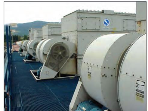
Centrifugal Fans with Inherently Low Sound Characteristics
