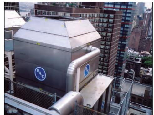
Intake and Discharge Sound Attenuation
