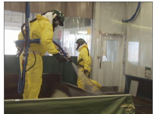
TriArmor® Corrosion Protection System Spray Booth
