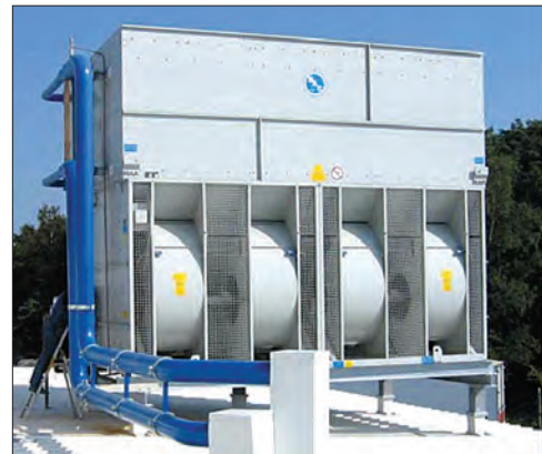
Closed Circuit Cooling Tower with the Optional Thermosetting Hybrid Polymer
