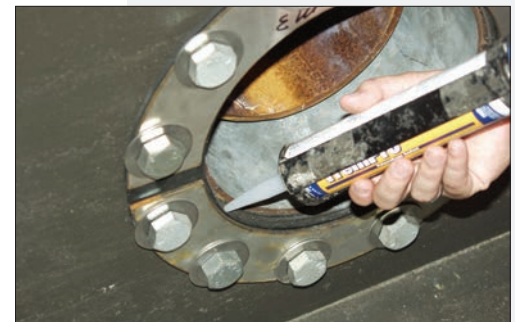
Figure 13. Caulk Exposed Galvanized Steel
