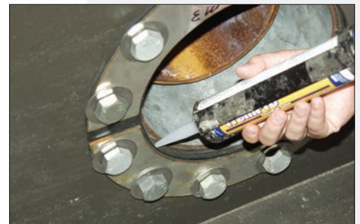
Figure 13. Caulk Exposed Galvanized Steel
