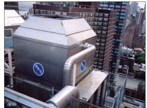
Intake and Discharge Sound Attenuation
