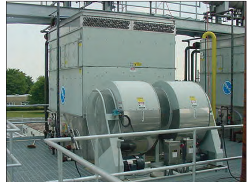
Standard VCL Construction Installation
