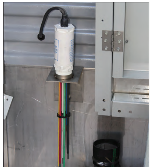
Electric Water Level Control
