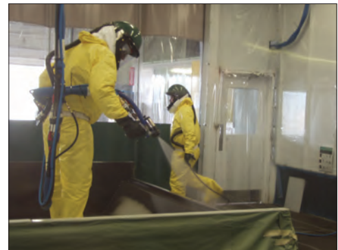
Application of TriArmor® Corrosion Protection System
