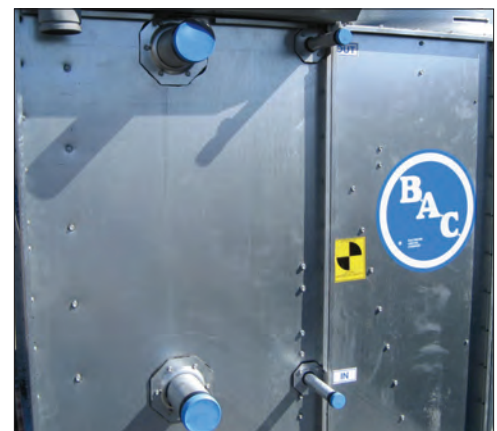
Multiple Circuit Coil
