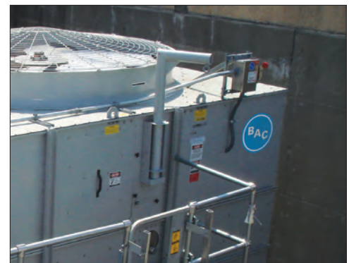
Motor Removal Davit Arm with Motor Removal Mount
