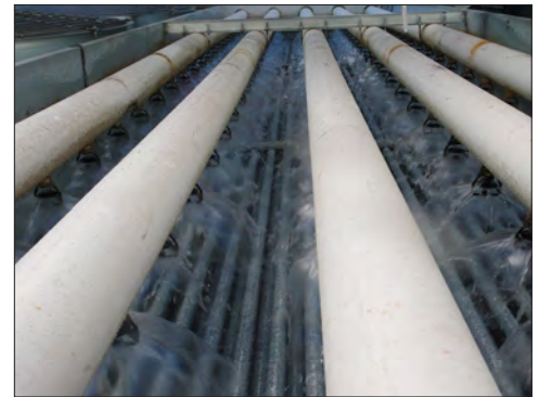
Spray Water Distribution System
