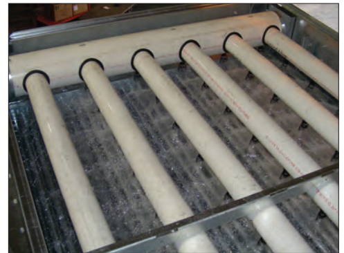
Spray Distribution For Easy Nozzle Inspection
