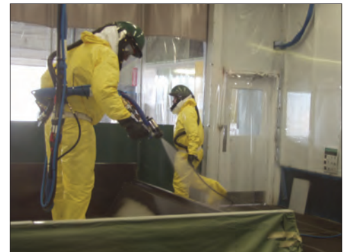
Application of TriArmor® Corrosion Protection System
