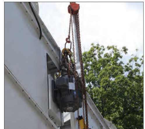
Motor Removal System
