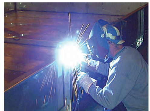
Welded Stainless Steel Basin
