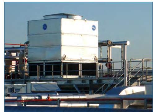
Rigging of Standard Construction Installation
