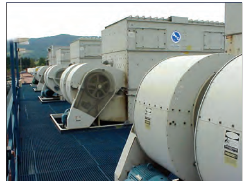
Centrifugal Fans with Inherently Low Sound Characteristics
