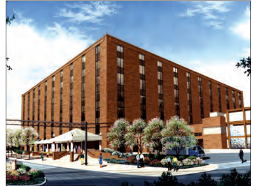
Friendship Annex 3 Office Building
