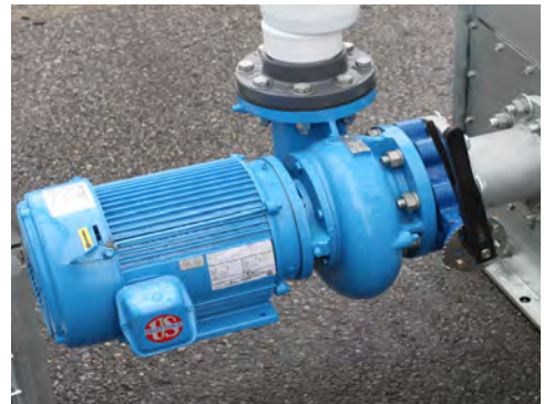
Spray Water Pump
