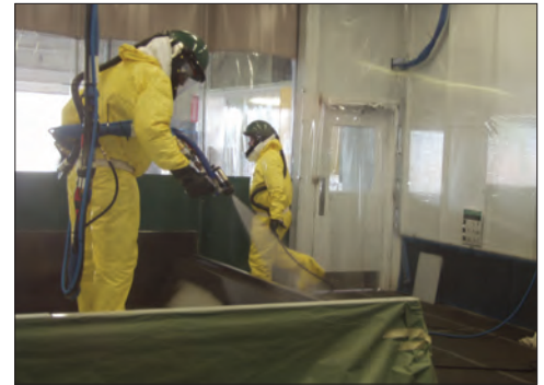
Application of TriArmor® Corrosion Protection System
