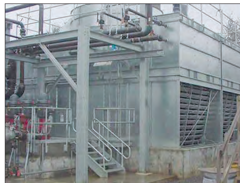
Basinless Unit Construction
