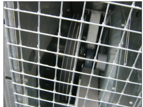
Air Intake Screens
