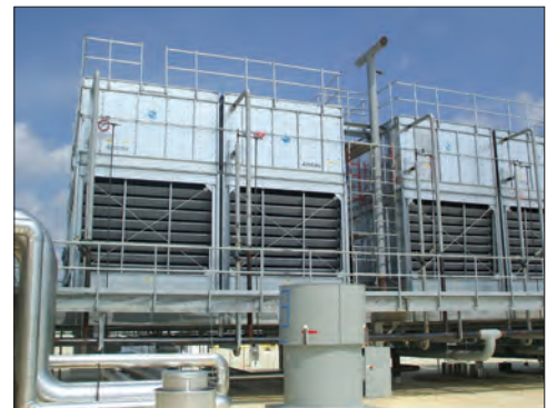
Multi-Cell CXVT Installation Showing Simplified Piping
