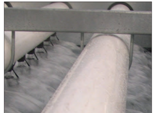
Non-clog Nozzles Ensure Even Flow Over Coil Area
