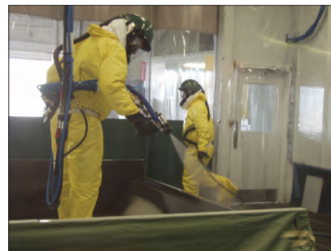
Application of TriArmor® Corrosion Protection System
