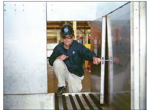
Internal Walkway with Large Access Door
