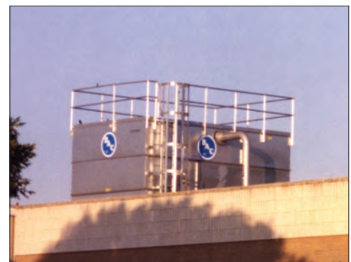
Handrails Packages and Ladders
