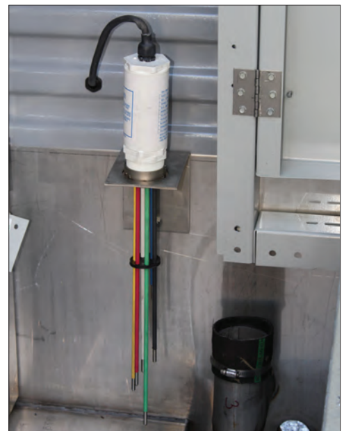
Electric Water Level Control
