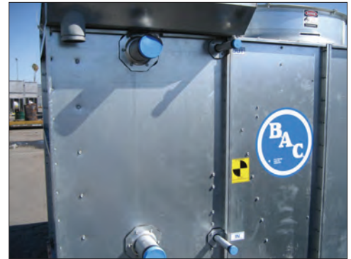
Multiple Circuit Coil
