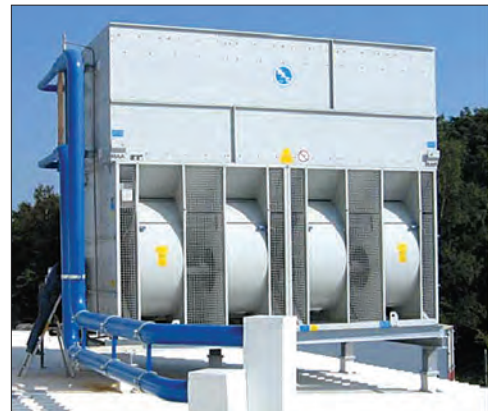
Closed Circuit Cooling Tower with the Optional Thermosetting Hybrid Polymer
