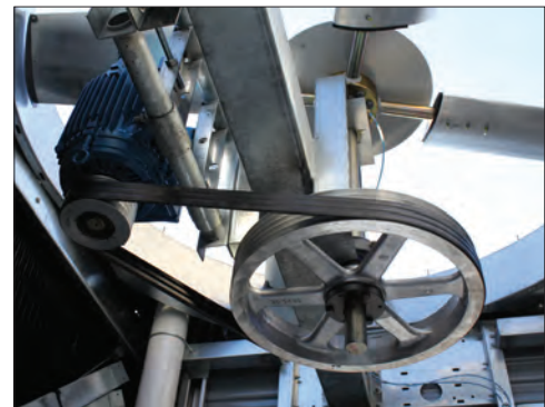
BALTIDRIVE® Power Train Fan System
