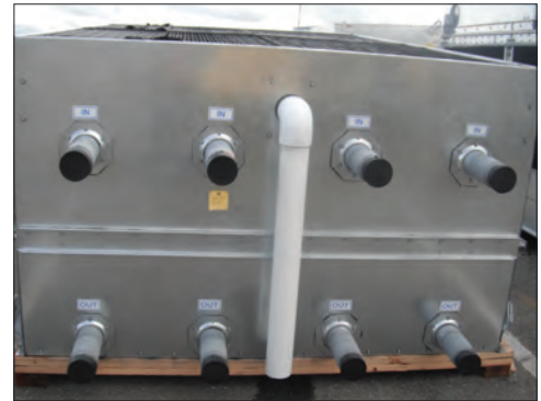
Multiple Circuit Coil Connections
