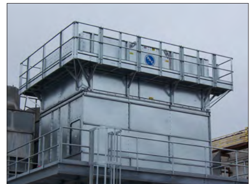
Pre-Assembled External Platform
