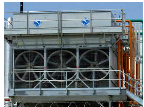
EVERTOUGH™ Construction Installation
