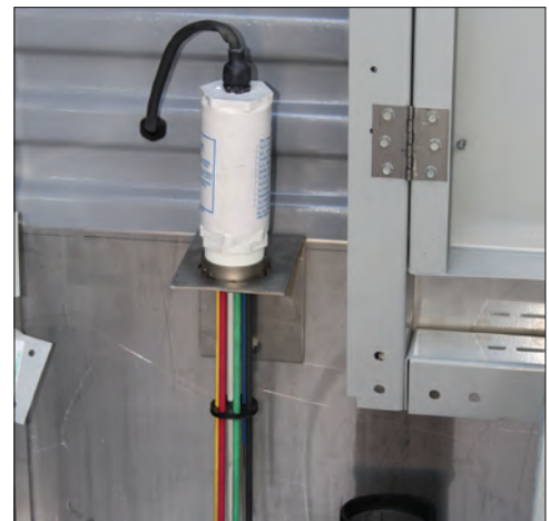
Electric Water Level Control
