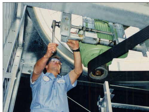
Figure 2. Adjustable Motor Base on Dual Air Intake FXV3/CXVT
