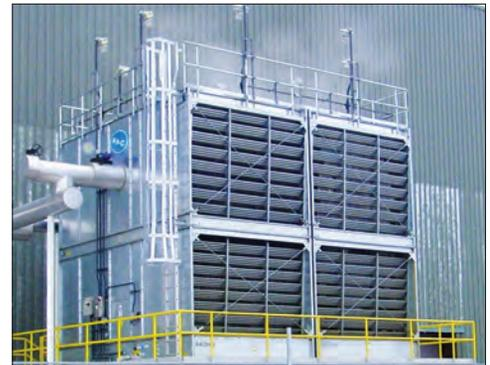
External Ladder, Safety Cage, and Handrail
