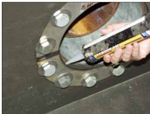
Figure 8. Caulk Exposed Galvanized Steel
