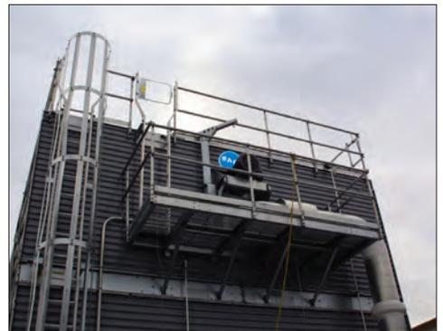
External Motor Platform, Ladder, Handrails, and Safety Cage
