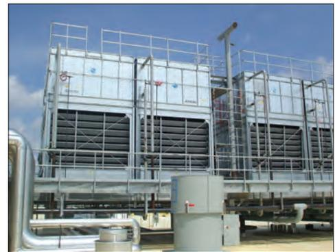
Multi-Cell CXVT Installation Showing Simplified Piping
