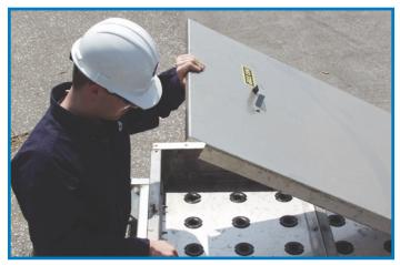
Any possible maintenance of the water distribution system can be further simplified with BAC's optional EASY CONNECT® Piping Arrangement with BAL-ANCE CLEAN® Chamber. The unique design of this exclusive BAC option allows any maintenance of the distribution basins to be performed from the interior of the tower, thereby eliminating the need to access the cooling tower fan deck to perform routine maintenance of the hot water distribution system.
