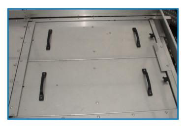
Series 3000 and Series 1500 Cooling Towers are equipped with easily removed steel hot water distribution basin covers as standard. Basin covers reduce maintenance requirements of the water distribution system by eliminating exposure of the entering water to airborne debris and sunlight, which reduces dirt accumulation and algae growth in the distribution basins. The distribution basin covers are constructed of the same rugged materials as the hot water basin.
