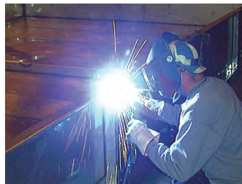
Welded Stainless Steel Cold Water Basin
