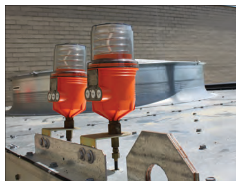
Automatic Bearing Greaser
