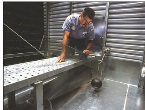
Mechanical Water Level Control
