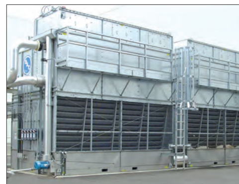
PCD Hood Installation
