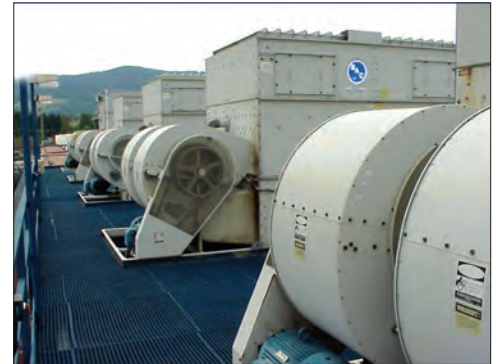
Centrifugal Fans with Inherently Low Sound Characteristics
