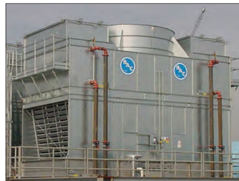
PCD Hood and External Platform
