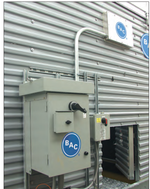
VFD with Pre-wired Terminal Box
