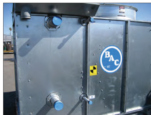
Multiple Circuit Coils
