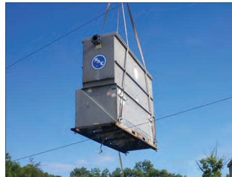
Single Piece Lift of a VTO Cooling Tower
