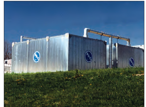
Modular Ice Thermal Storage Unit
