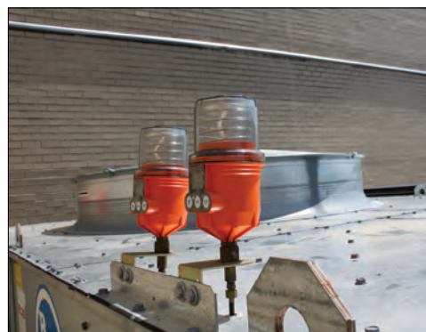
Automatic Bearing Greasers
