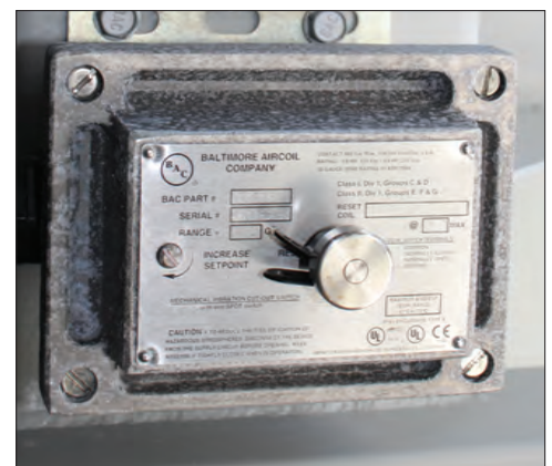
Vibration Cutoff Switch
