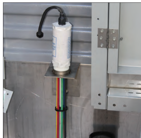
Electric Water Level Control
