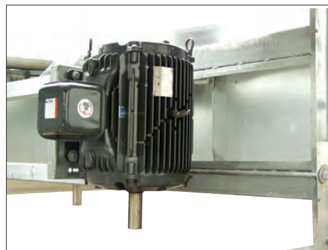
BALTDRIIVE® Power Train Internally Mounted Motor Models PT2-1009A, PT2-1012A, PT2-1212A, and PT2-1218A
