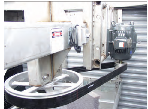
BALTIDRIVE® Power Train Fan System
