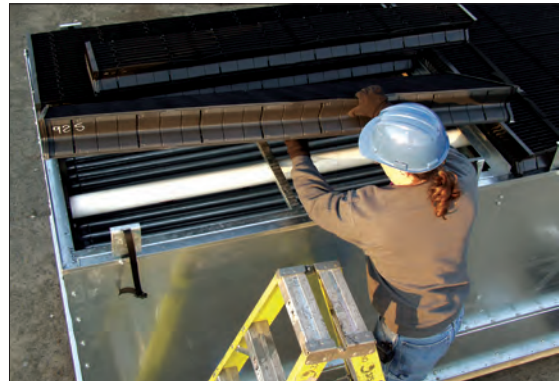
Inspecting Drift Eliminator
