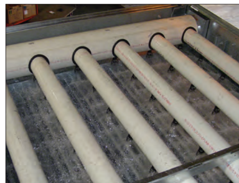
Operating Spray Distribution System
