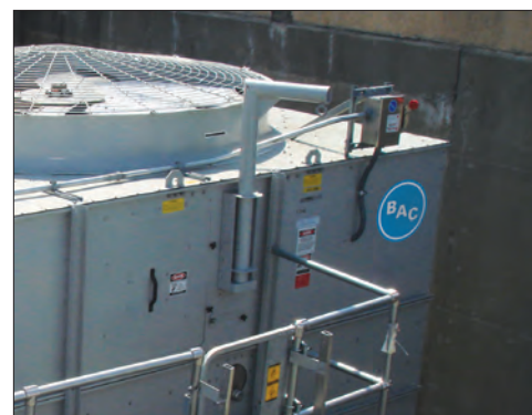
Motor Removal Davit Arm with Motor Removal Mount
