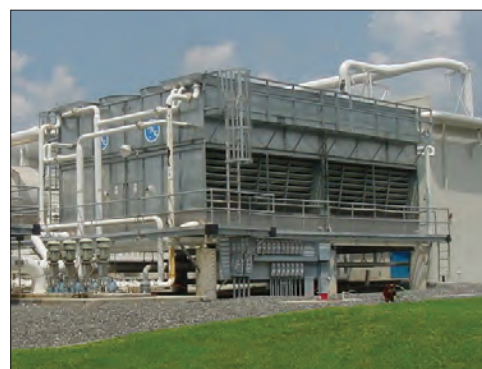
All Steel Panel Construction
