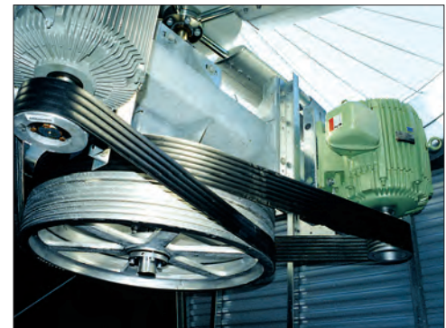
BALTIGUARD™ Fan System Provides Built in Redundancy
