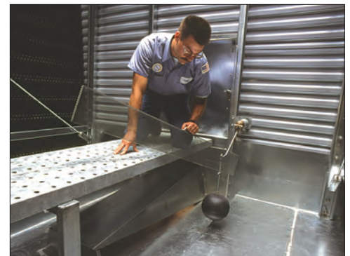
Mechanical Water Level Control
