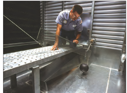
Mechanical Water Level Control
