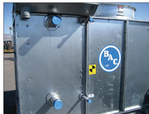
Multiple Circuit Coils
