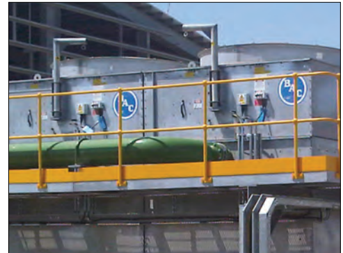
Motor Removal System with Davit Arms
