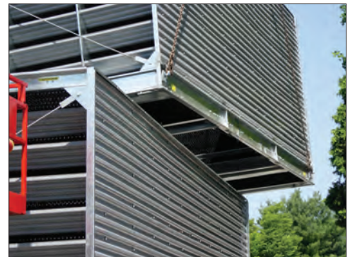
Rigging Guides Ensure Alignment
