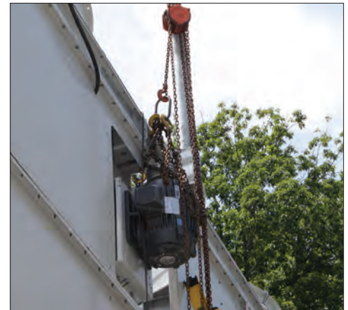
Motor Removal System
