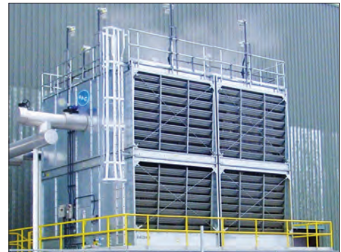
External Ladder, Safety Cage, and Handrail
