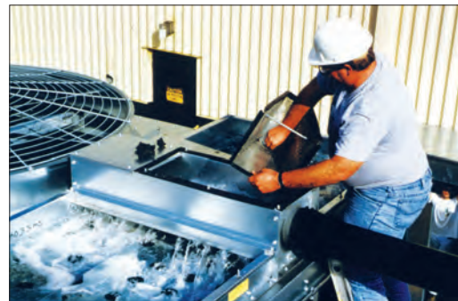
Hot Water Basin Strainer Cleaning (Series 1500 Cooling Towers Only)
