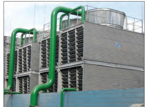
Velocity Recovery (VR) Stacks
