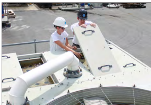
Gravity Water Distribution
