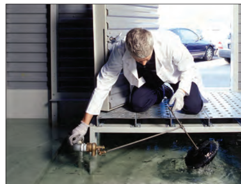
Mechanical Water Level Control
