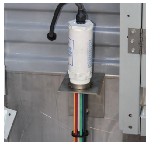
Electric Water Level Control
