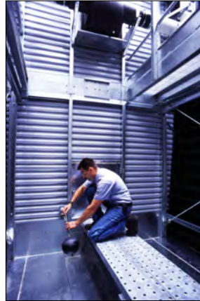
Mechanical Water Level Control
