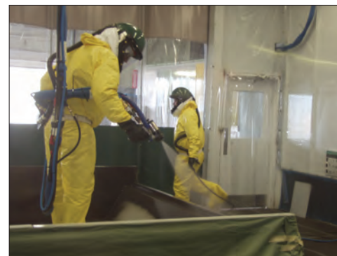
Application of TriArmor® Corrosion Protection System
