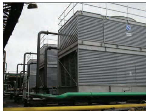
Standard FRP Casing Panels
