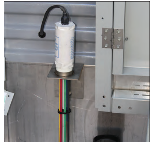
Electric Water Level Control
