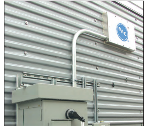
Series 3000 Terminal Box with Factory Wiring
