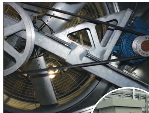
BALTIDRIVE® Power Train Used for VFD Applications
