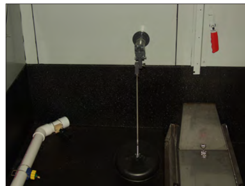
Mechanical Water Level Control
