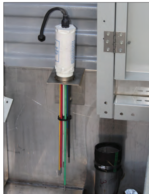
Electric Water Level Control
