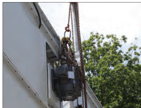
Motor Removal System
