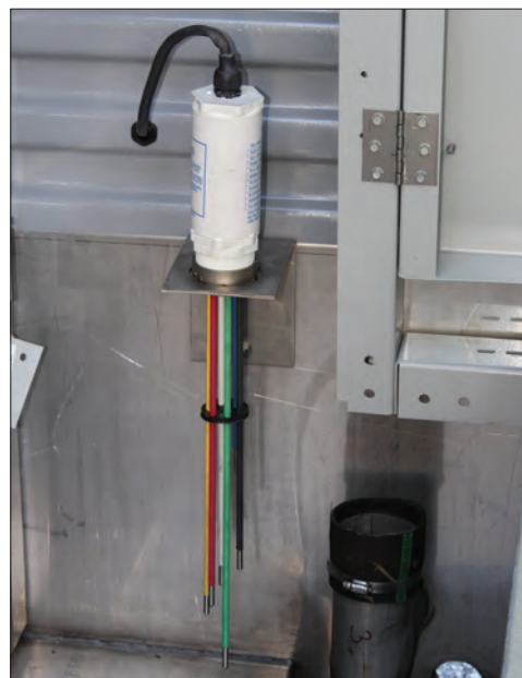
Electric Water Level Control
