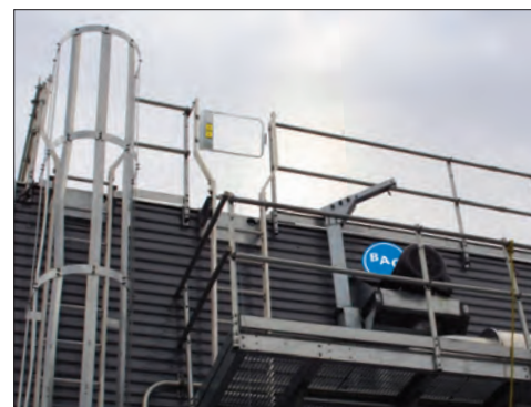
Motor Removal System with Davit Arm, Motor Access Platform, and Handrail Package
