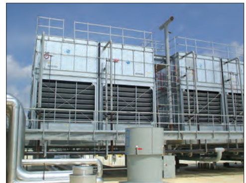
Multi-Cell CXVT Installation Showing Simplified Piping
