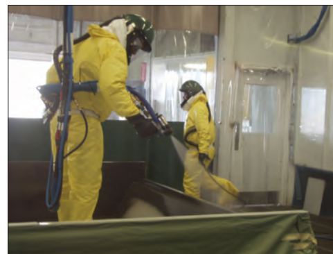
Application of TriArmor® Corrosion Protection System
