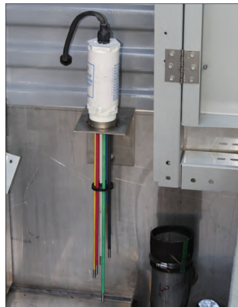
Electric Water Level Control
