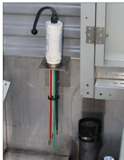
Electric Water Level Control
