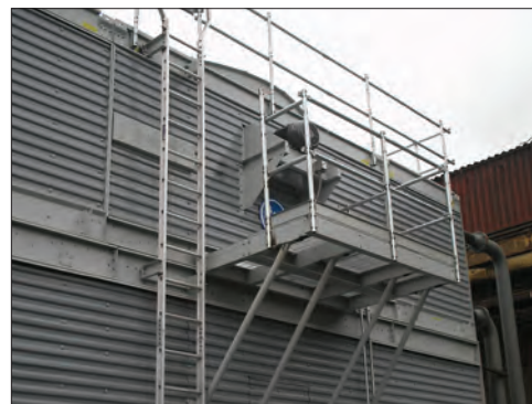
External Motor Platform
