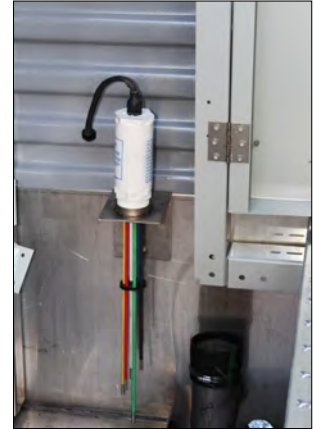
Electric Water Level Control
