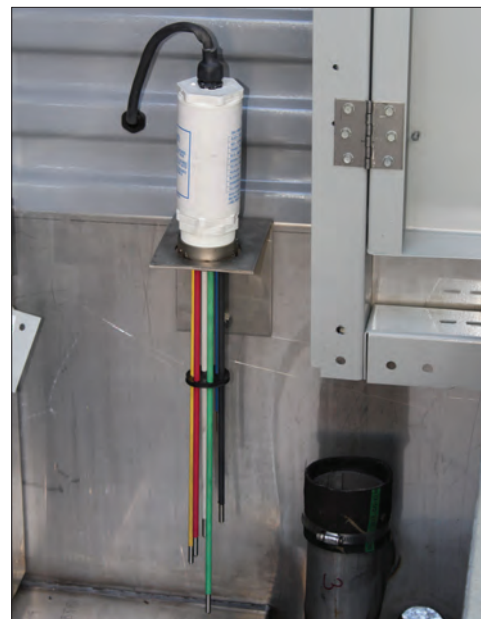
Electric Water Level Control
