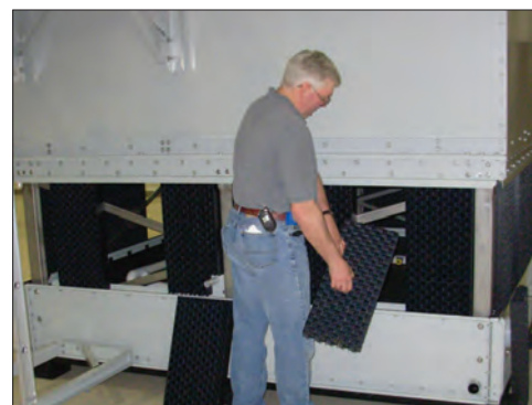
Combined Inlet Shields
