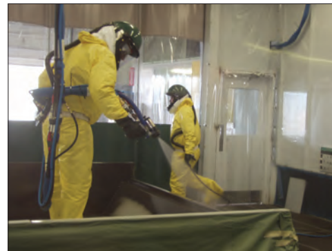
Application of TriArmor® Corrosion Protection System
