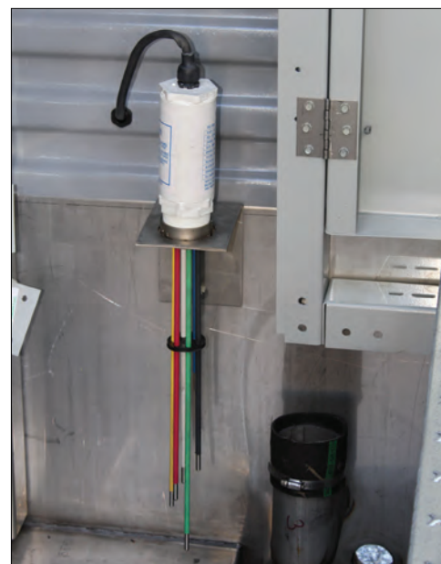
Electric Water Level Control
