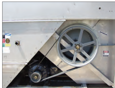
BALTIDRIVE® Power Train Fan System
