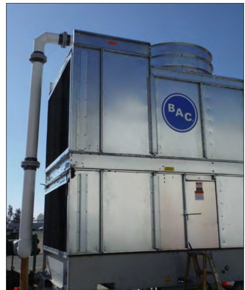
Standard Single Inlet Connection
