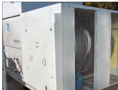
Intake Sound Attenuation
