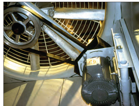
BALTIDRIVE® Power Train Fan System
