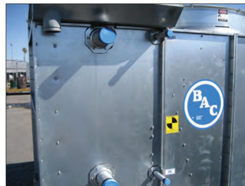
Multiple Circuit Coil
