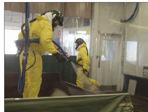
Application of TriArmor® Corrosion Protection System
