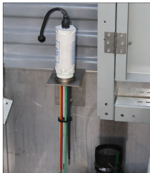
Electric Water Level Control
