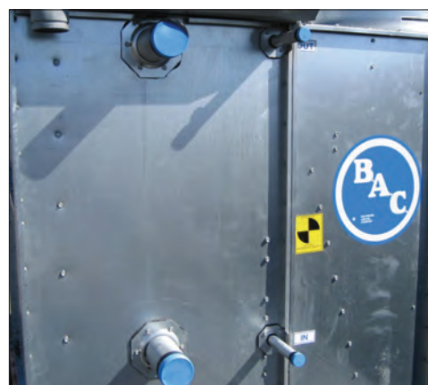
Multiple Circuit Coil
