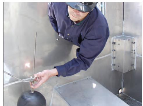
Standard Mechanical Water Level Control
