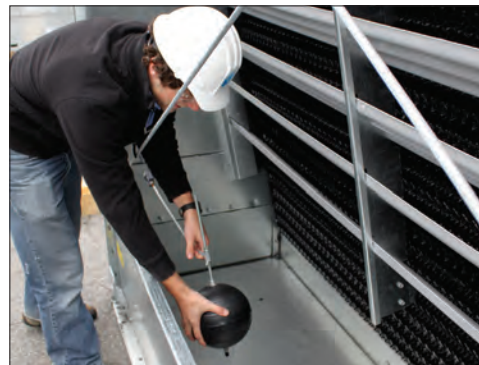
Mechanical Water Level Control
