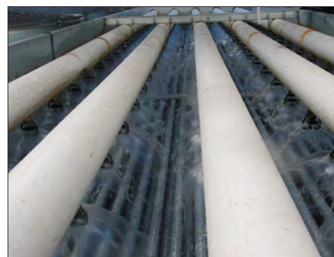
Spray Water Distribution System
