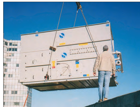
Single Piece Lift of a VFL
