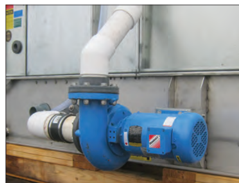
Standard Spray Water Pump
