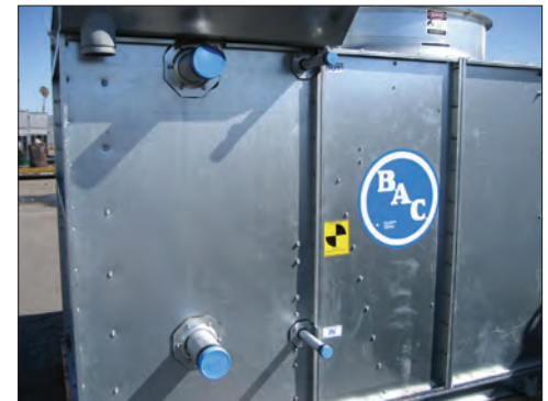
Multiple Circuit Coil
