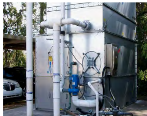
Standard Spray Water Pump
