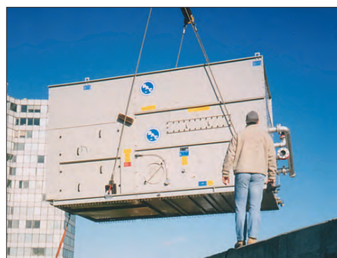
Single Piece Lift of a VFL
