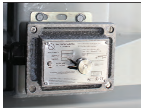
Vibration Cutoff Switch
