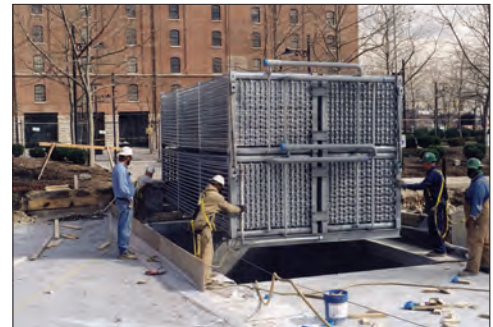
BAC ICE Coil Installation Camden Yards
