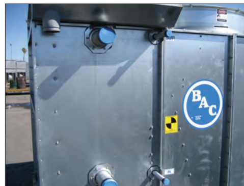
Multiple Circuit Coil
