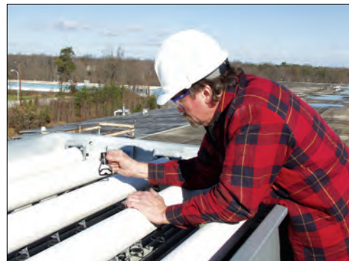
Inspecting Spray Nozzles
