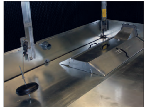
Mechanical Water Level Control
