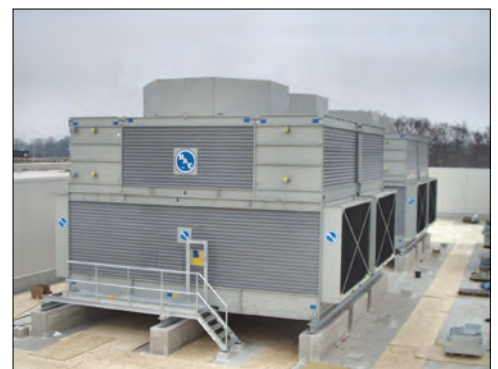
An Evaporative Condenser with Full Sound Attenuation
