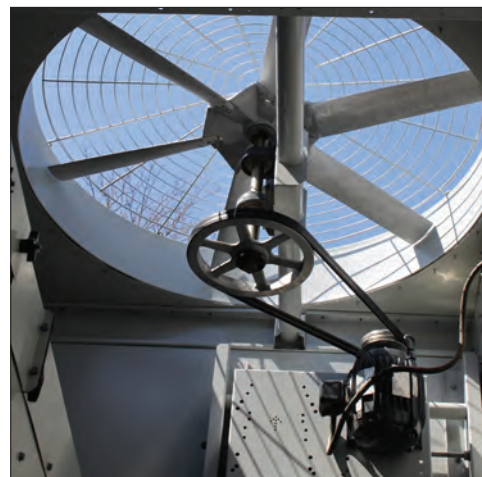
BALTIDRIVE® Power Train Fan System
