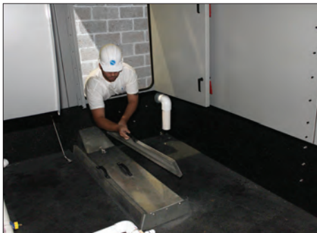
Inspecting a Cold Water Basin Strainer
