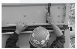
Figure 5. Drift Pin Alignment
