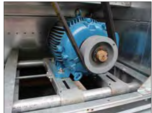
BALTIDRIVE® Power Train-Upgraded Motor Base
