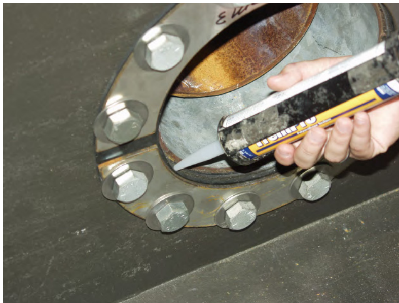
Figure 100. Caulk Exposed Galvanized Steel
