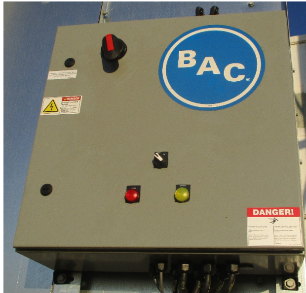
Figure 22. EC Fan Control Enclosure for Models VRC-xxxxA-xxxxN-xB
