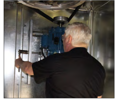
Figure 3. Adjustable Motor Base
