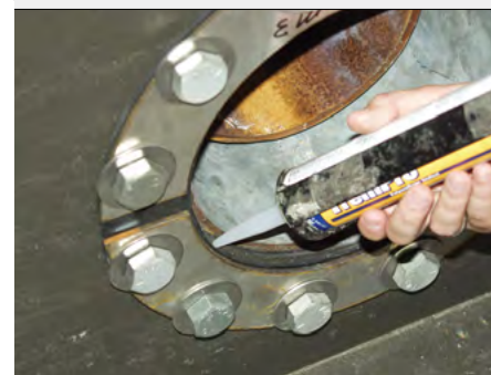
Figure 14. Caulk Exposed Galvanized Steel
