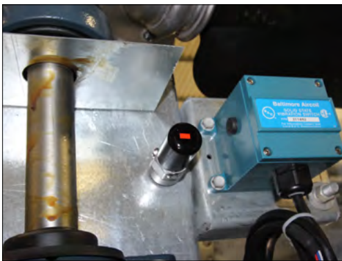
Figure 11a. Preferred Accelerometer Location
