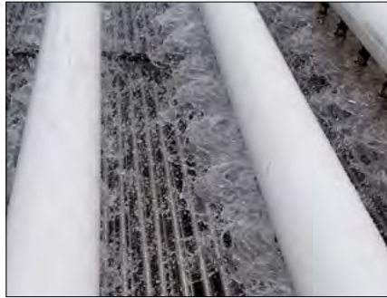
Figure 7. Nozzle Spray Pattern
