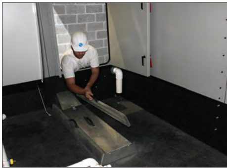
Inspecting a Cold Water Basin Strainer
