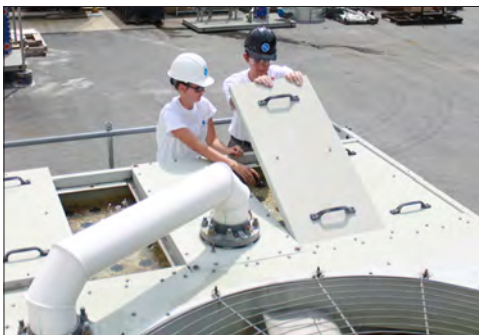
Gravity Water Distribution
