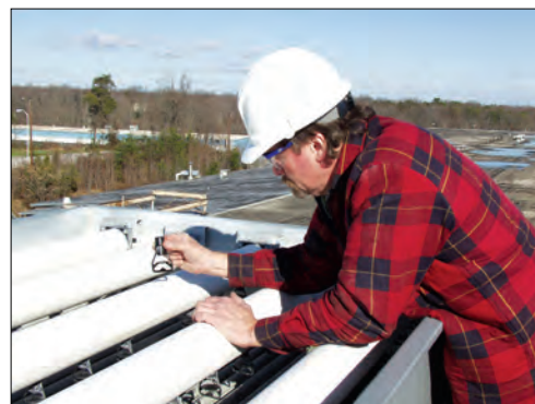
Inspecting Spray Nozzles
