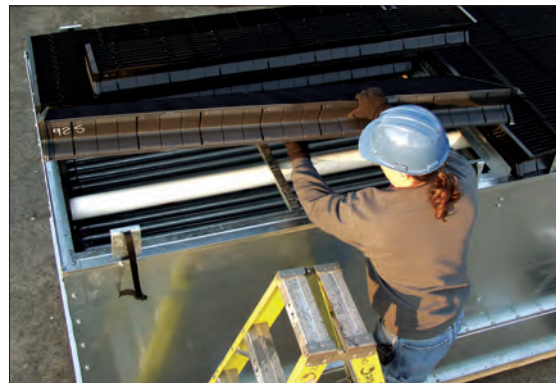
Inspecting Drift Eliminator
