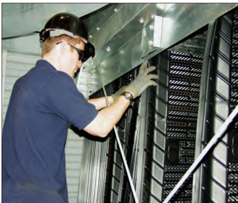
Installing Retrofit VersaCross Fill Kit
