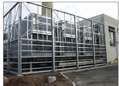
Barrier Walls Being Erected Around FXV Dual Air Intake Units
