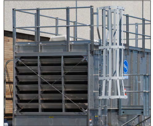
External Ladder and Platform
