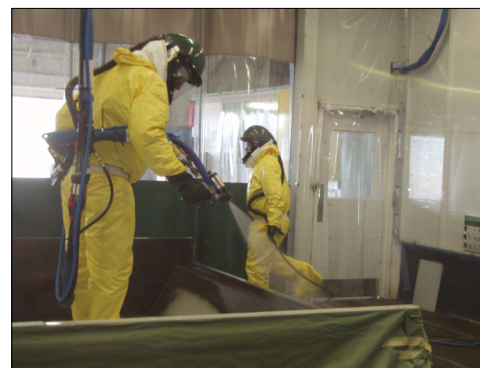
Application of TriArmor® Corrosion Protection System
