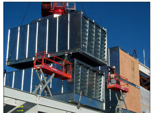
Rigging Guides Ensure Alignment
