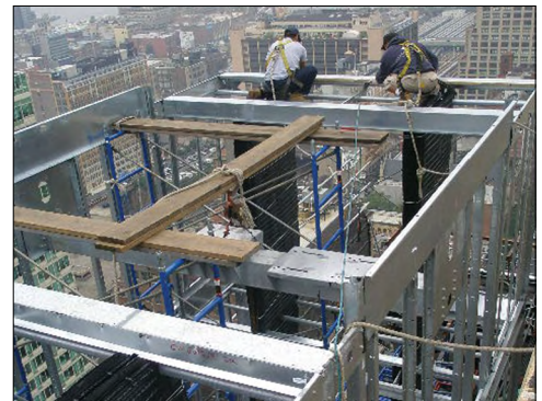
Knockdown Unit Installation
