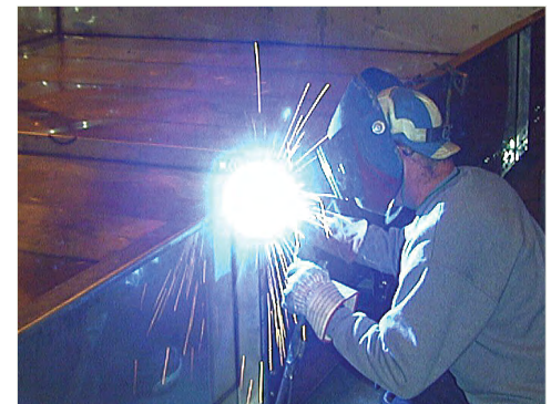
Welded Stainless Steel Cold Water Basin
