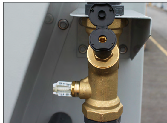
Figure 20b. Schematic for Water Flow Adjustment Screw
