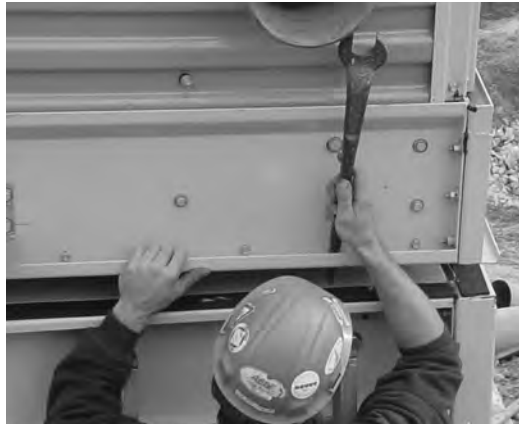
Figure 5. Drift Pin Alignment
