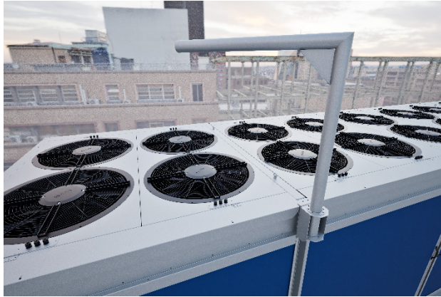
Figure 25: Fan Removal System
