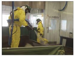
Application of TriArmor® Corrosion Protection System
